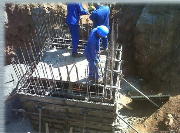
Concrete Casting: Pump Station Kuruman Housing Project
