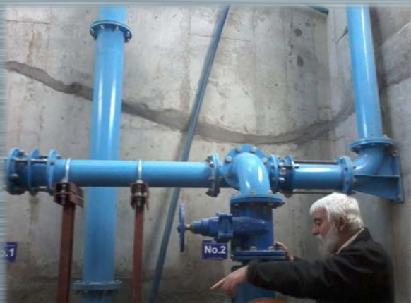
Greenpoint Pump Station
