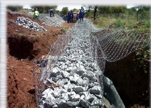
Gabion Cages, Kuruman
